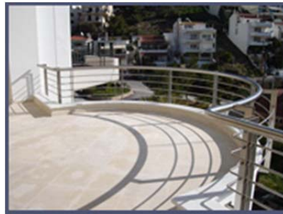
Balustrades of Balconies
