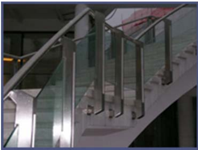
Balustrades of Stairs
